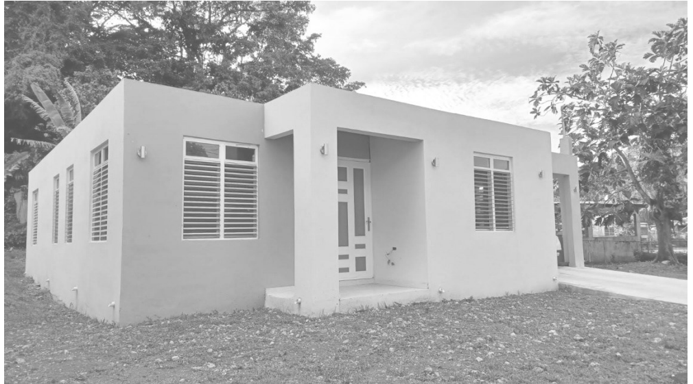
Mayra Salgado's "newly" constructed house in Puerto Rico showing the windows and front door made possible with donations from St Peter's.
